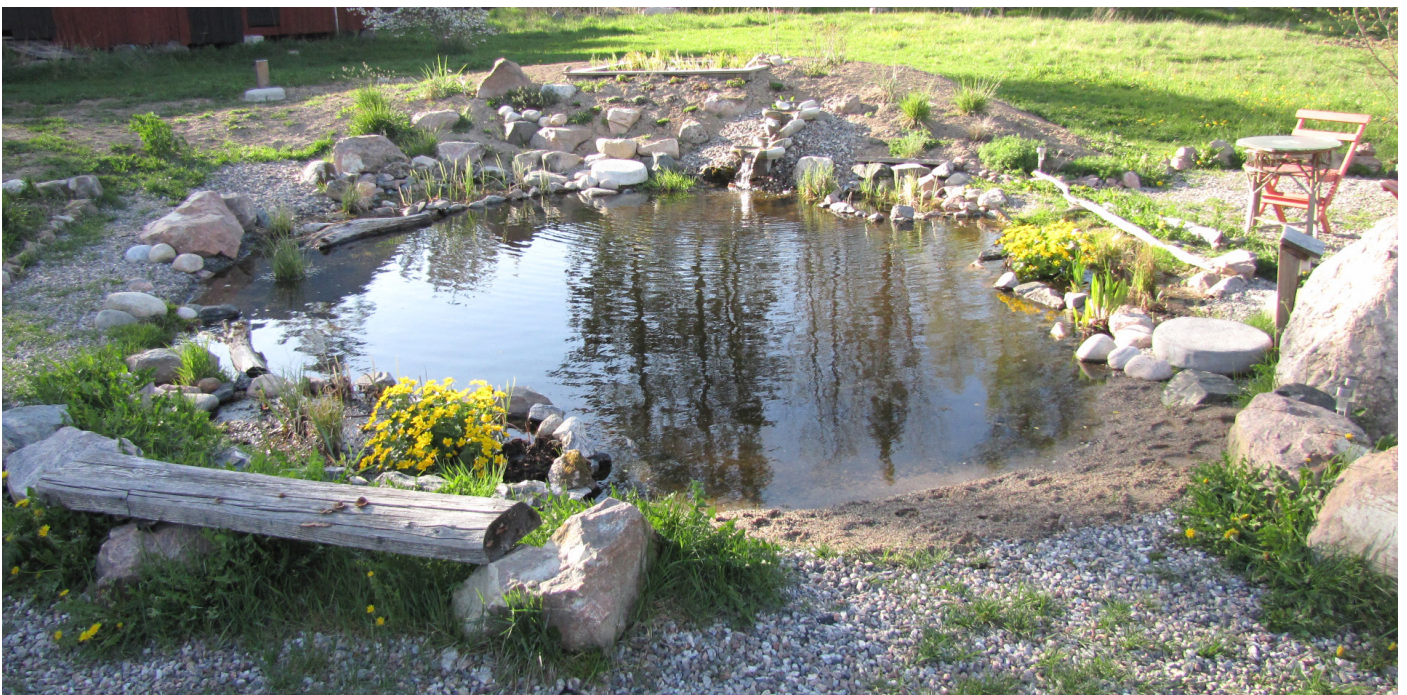
'Greywater dam' – a constructed wetland – where wastewater purification works through green phytotechnology. Seen in the background is the first step where the sludge in the greywater is composted in a reed bed; followed by the second step in the front where the separated greywater is recycled in a pond with plants via a water ladder for oxygenation.
